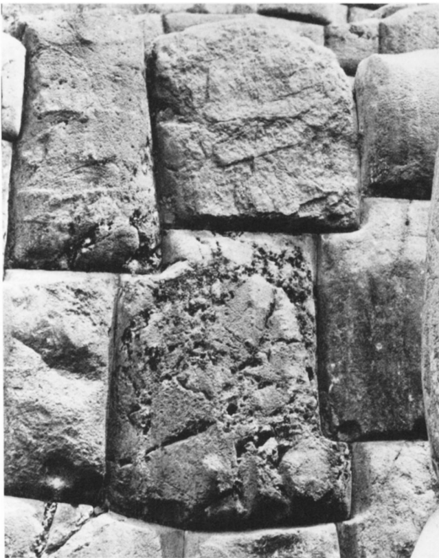
Fig. 35. Illustration of the combined effect of the fitting of bedding joints and lateral joints at Saqsaywaman.
