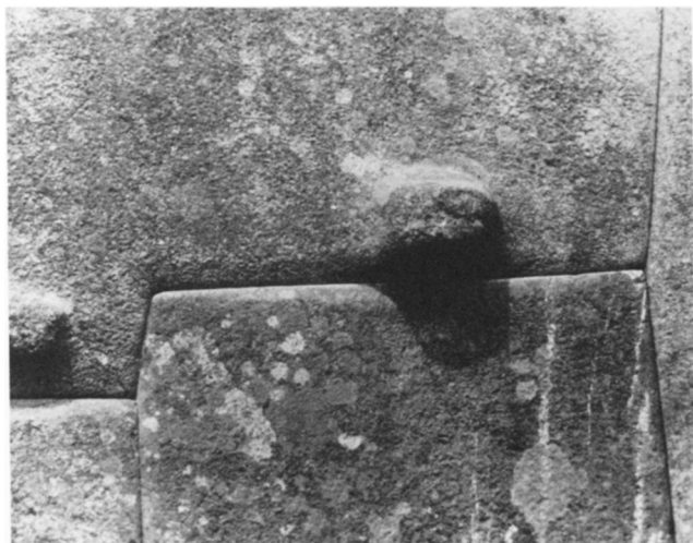
Fig. 28. Exception to bedding-joint rule at Ollantaytambo.
