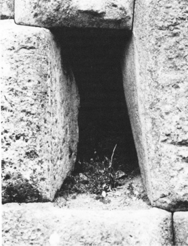
Fig. 38. Gap left by a keystone fallen out of bond. Notice taper of the sides of the gap leaving a wedge-like hole. Since the width of the hole is wider at the bottom than at the top, the keystone must have been introduced from the front.
